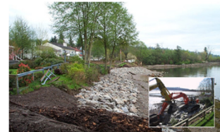
Erosion protection, Dollarton foreshore, North Vancouver, BC
